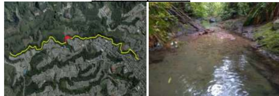
Colector Zanjón Hondo
